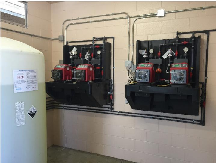
**Figure 3. Two packaged pump systems that were manufactured so they can be wall mounted to conserve space. These systems have manifold, gauges, pressure relief, safety shut-off valves and the base of the unit functions as spill containment.**
