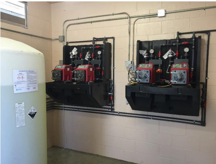
*Figure 3. Two packaged pump systems that were manufactured so they can be wall mounted to conserve space. These systems have manifold, gauges, pressure relief, safety shut-off valves and the base of the unit functions as spill containment.*
